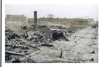
The boardwalk fire burned everything from Moorlyn Terrace to 10th street. In this picture you can see the burnt wooden pilings in the ground. Later, the new wooden boardwalk was built with cement pilings.
